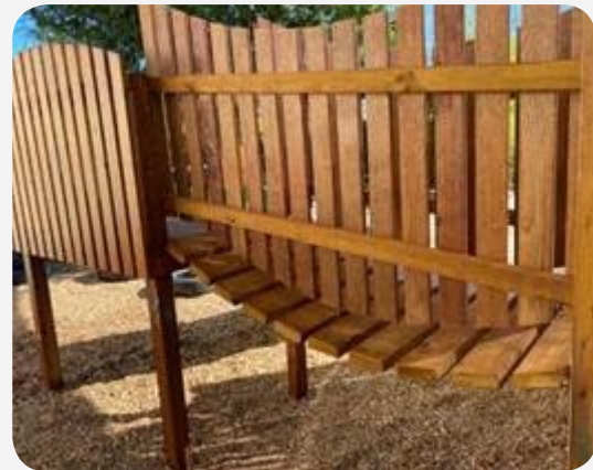
Before and after: The rope bridge was changed to a wooden bridge, ensuring all children can access and enjoy the equipment safely and confidently, and move freely through each area with their peers.
